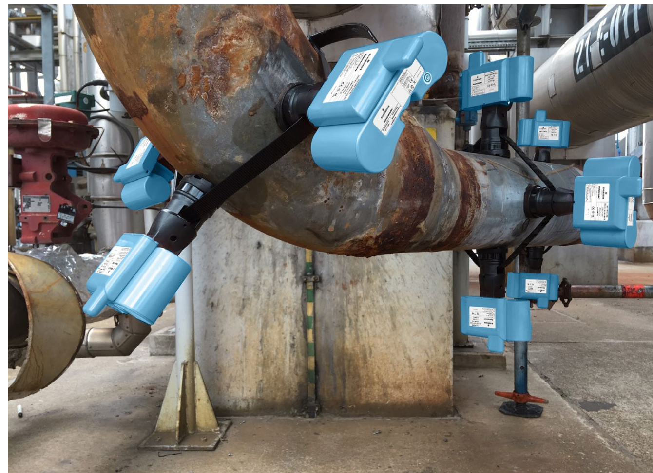
FIGURE 5 If process changes might increase the risk of corrosion or erosion, monitoring wall thickness using Rosemount Wireless Corrosion and Erosion Transmitters can warn of developing containment issues.
